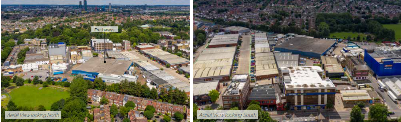
Figure 2: Aerial View of Existing Site
