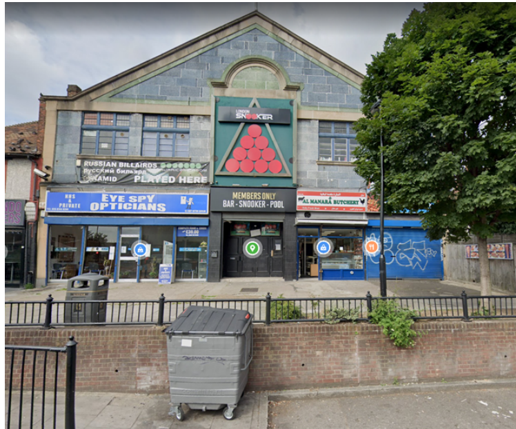
Figure 2: Existing Site Frontage
