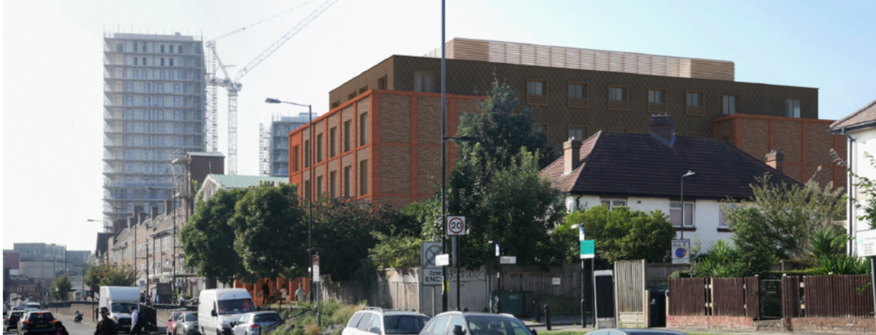
Figure 7: Street Scene with Argos Homebase Superstore Development Under Construction
